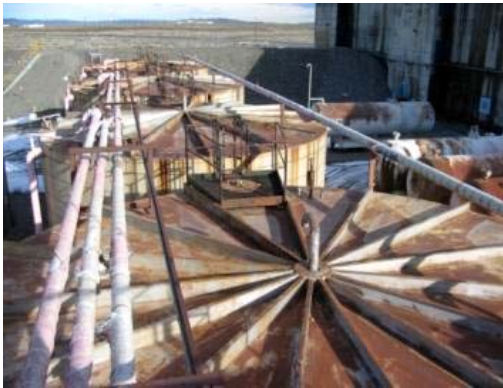
Vertical tanks near the Hanford Site's U Plant before (left) and after (right) asbestos thermal system insulation removed.
